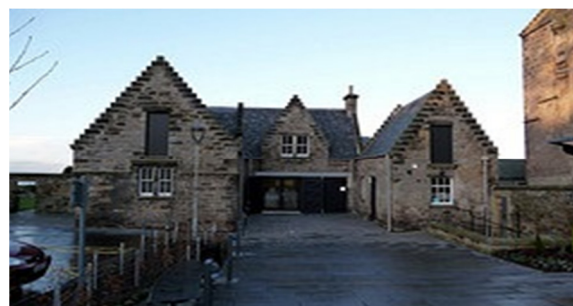
Museum Building where Tadpole was installed
